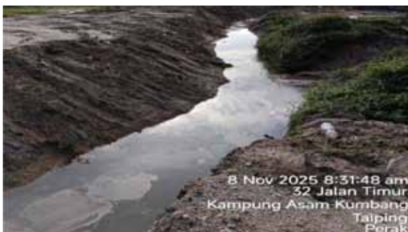
Drainage to guide water runoff away from access road and into water catchment pond. This is done to prevent muddy roads and cause less pollution.
