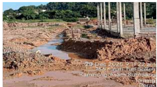
Drainage to guide water runoff away from access road and into water catchment pond. This is done to prevent muddy roads and cause less pollution.
