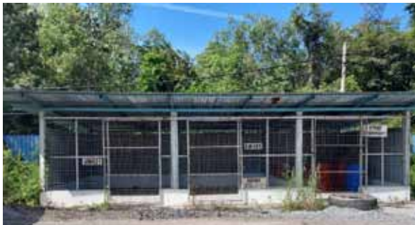
Scheduled waste storage at Pokok Sena, Kedah
