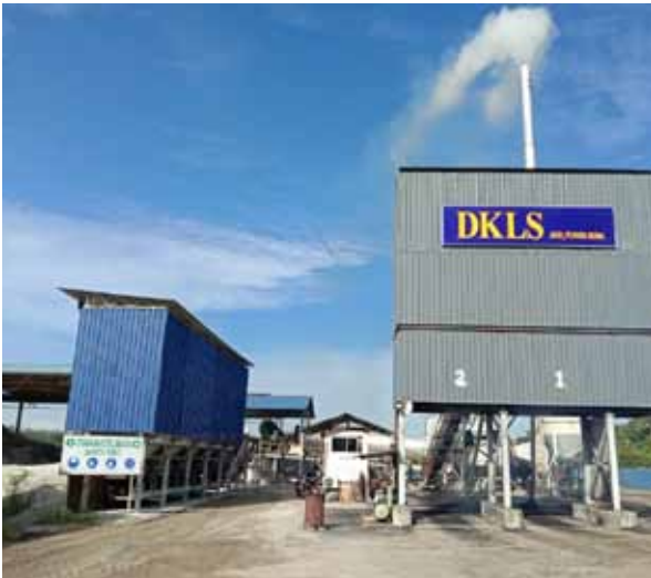
Premix Plant at Pokok Sena, Kedah
