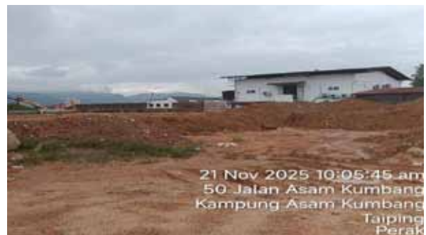
Stockpile have been levelled so that it is not affected or damaged by rain or wind.
