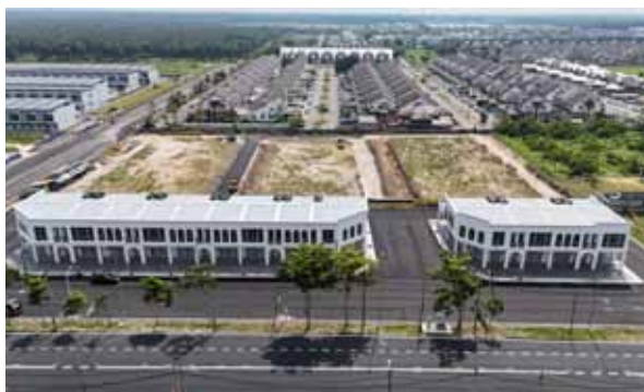
Double-storey shophouses at Kairos Commercial Square in Sitiawan, Perak
