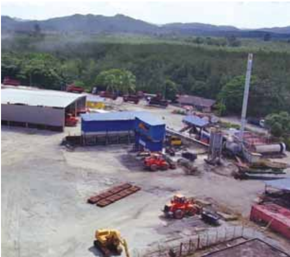
Premix Plant at Bukit Perak, Kedah
