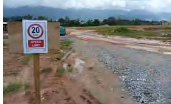
Visible speed limit signages (20km/h) are placed on sites. Low speed minimises dust flyoff.
