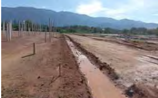
Drainage to guide water runoff away from access road. Prevents muddy roads, lesser pollution.
