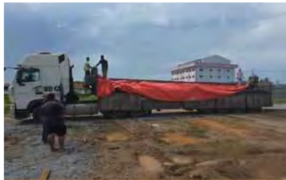
Lorries transporting construction materials are covered with canvas to reduce particles flying into the air.
